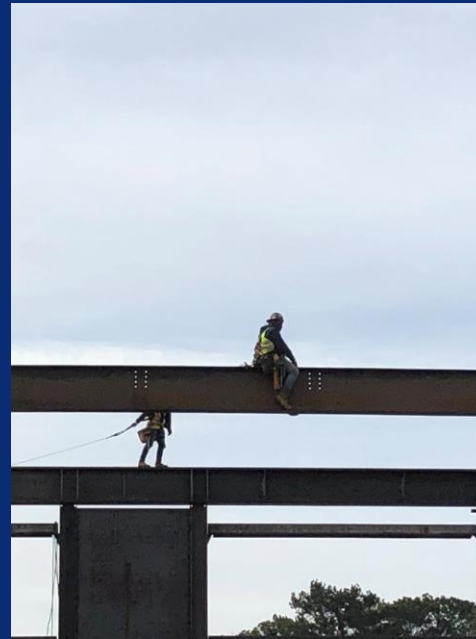
Iron workers installing sequence 1 & 2 steel
