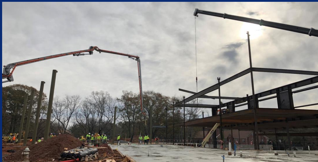
Photo of the project site with simultaneous concrete pour and steel install
