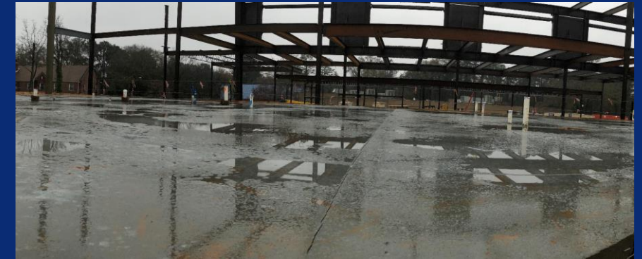
Main level west slab on grade poured
