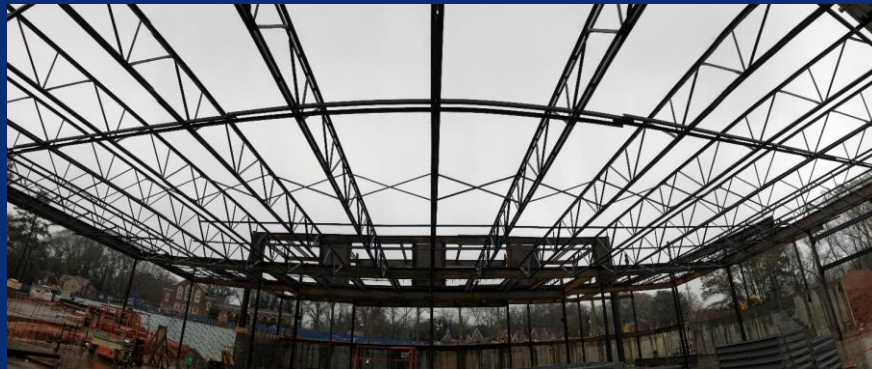
Bar joists installed over cafeteria
