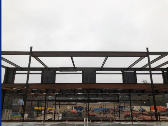
Transfer truss spanning gym installed
