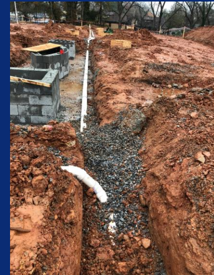
Sanitary lines for main level east installed
